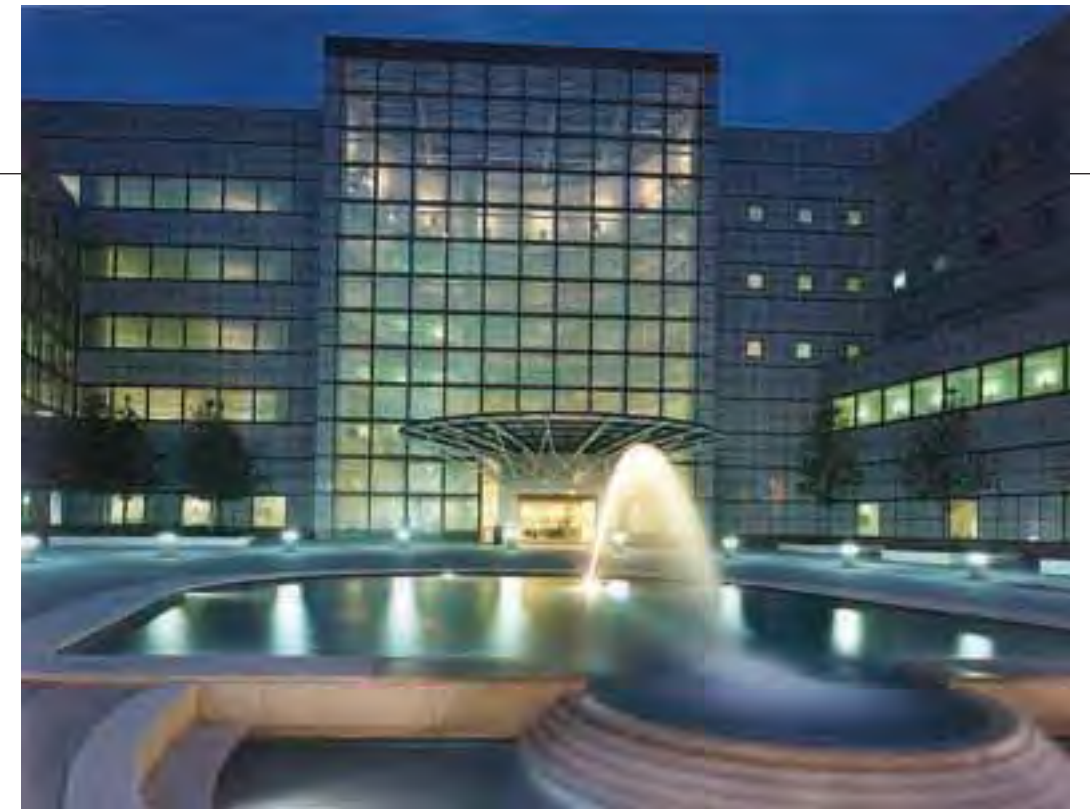
Constructed by Brasfield & Gorrie and designed by world renowned architect I. M. Pei, the center of Birmingham's Kirkland Clinic features a six-story concrete frame structure with two mechanical mezzanine levels.
