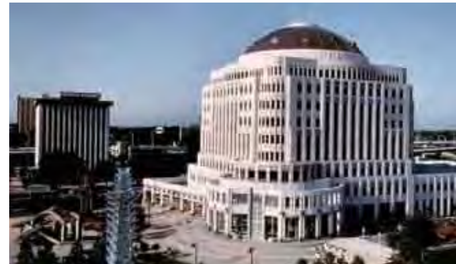
Constructed in 1992 by Brasfield & Gorrie, Orlando City Hall features contemporary architecture with Roman Revival elements.
